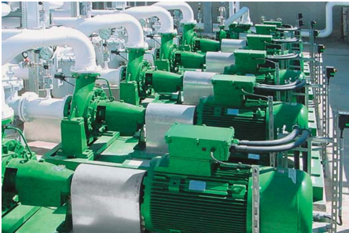
Type NCR acc. to API 610 with single mechanical seal. Liquid: Aviation fuel JP4.
