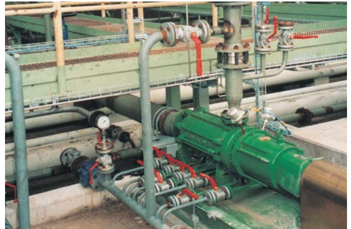
Type HZMR with magnetic coupling. Liquid: Benzol mixture.
