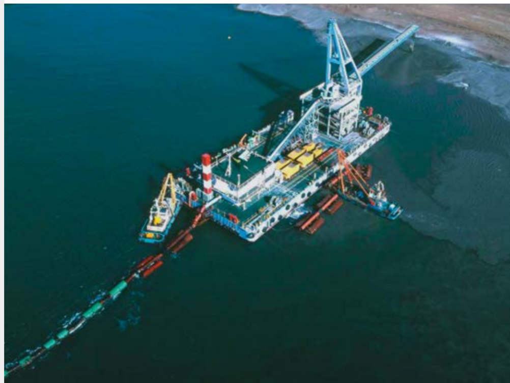
On the Japanese coast line, three huge KOS 25100 and 25200 piston pumps are pumping silt out of the sea for land reclamation. The Nagoya is now located on this new artificial island.
