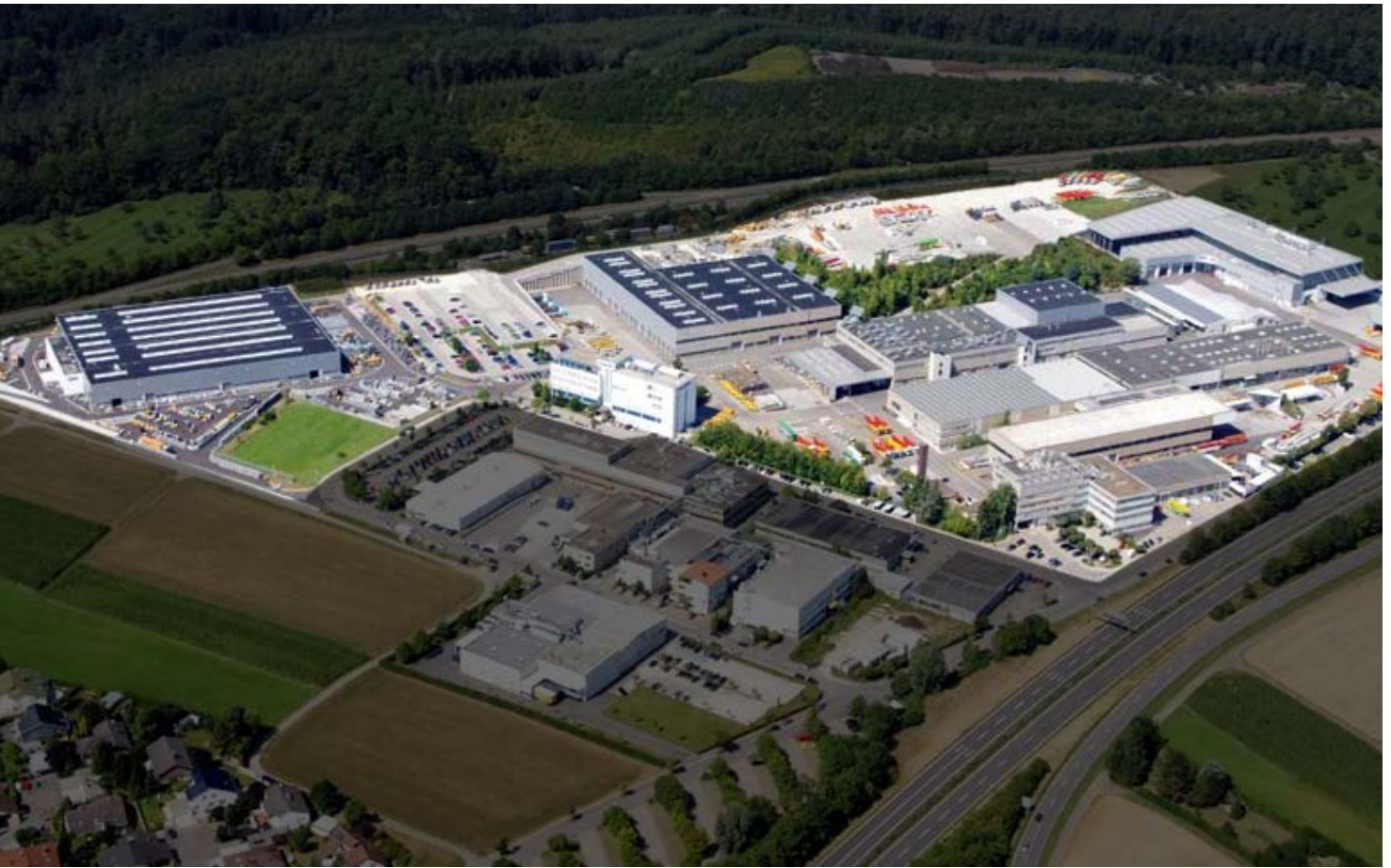
Putzmeister headquarter in Aichtal
