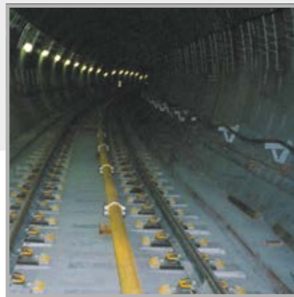
Safe laying of horizontal delivery lines with Zentrifix®
