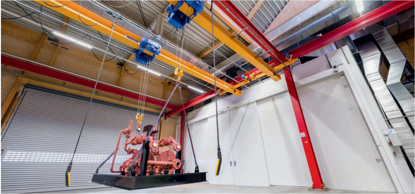
There are sufficient cranes for handling the modules.
